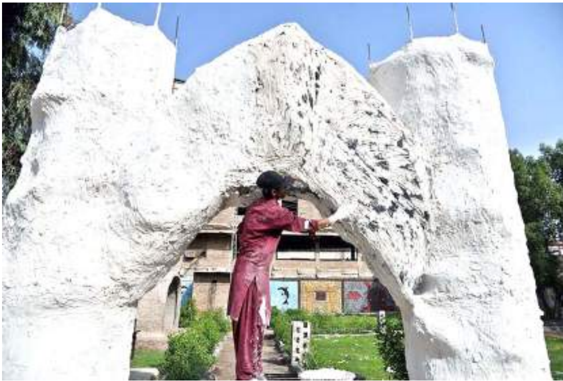
A worker is busy beautifying the entrance gate of the railway station park in an unconventional style.
