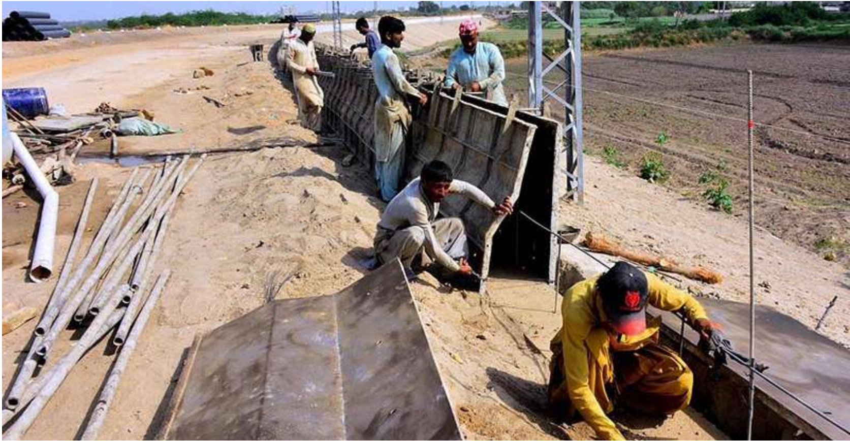
Labourers work on the construction of an embankment wall along the Indus River at Latifabad Unit No. 4 as part of a development project aimed at protecting local communities
