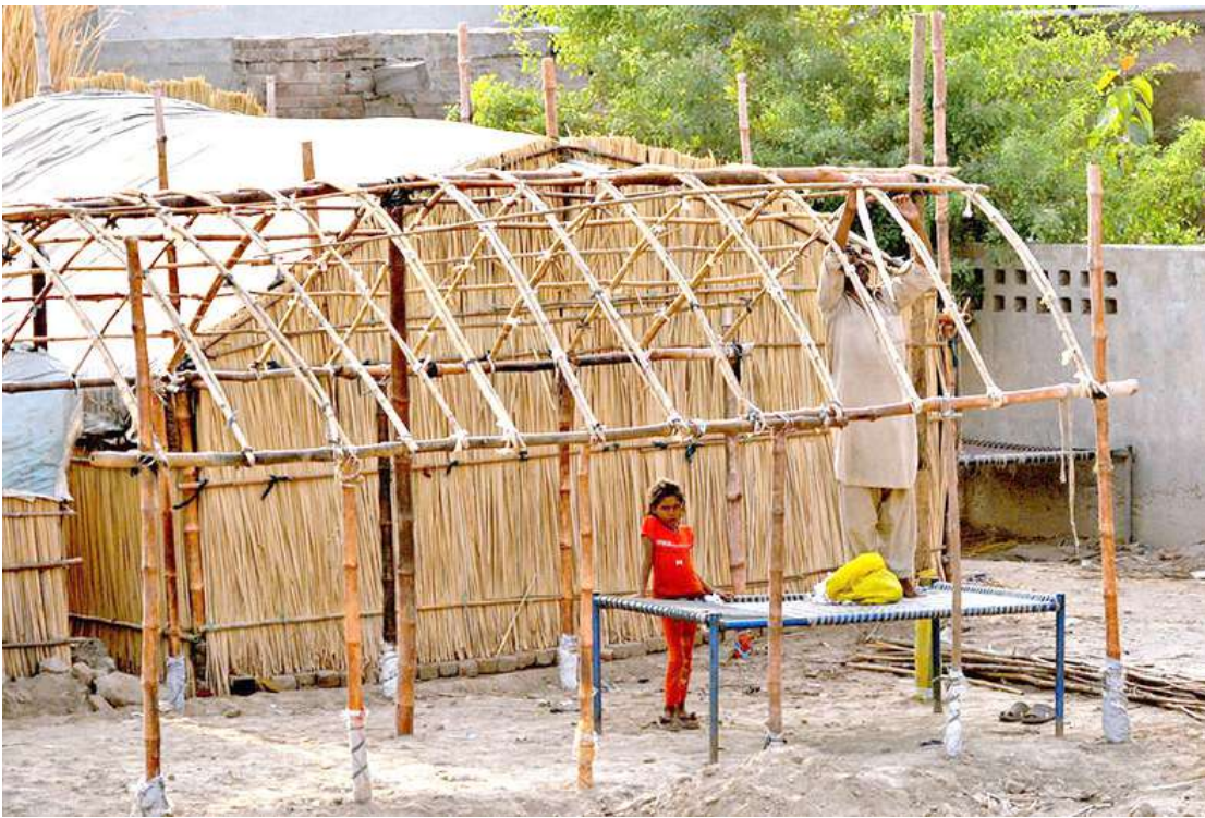
A man is constructing a makeshift shelter for his family using bamboo poles and reeds
