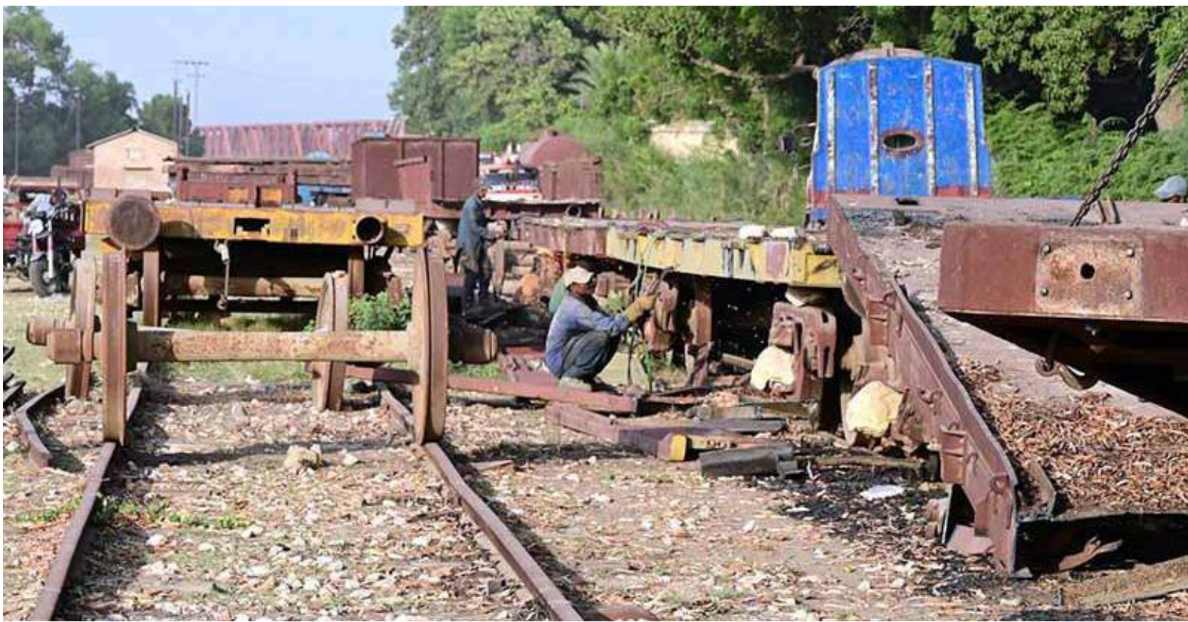
Railway workers are busy welding while repairing a goods train at Kotri Railway Workshop
