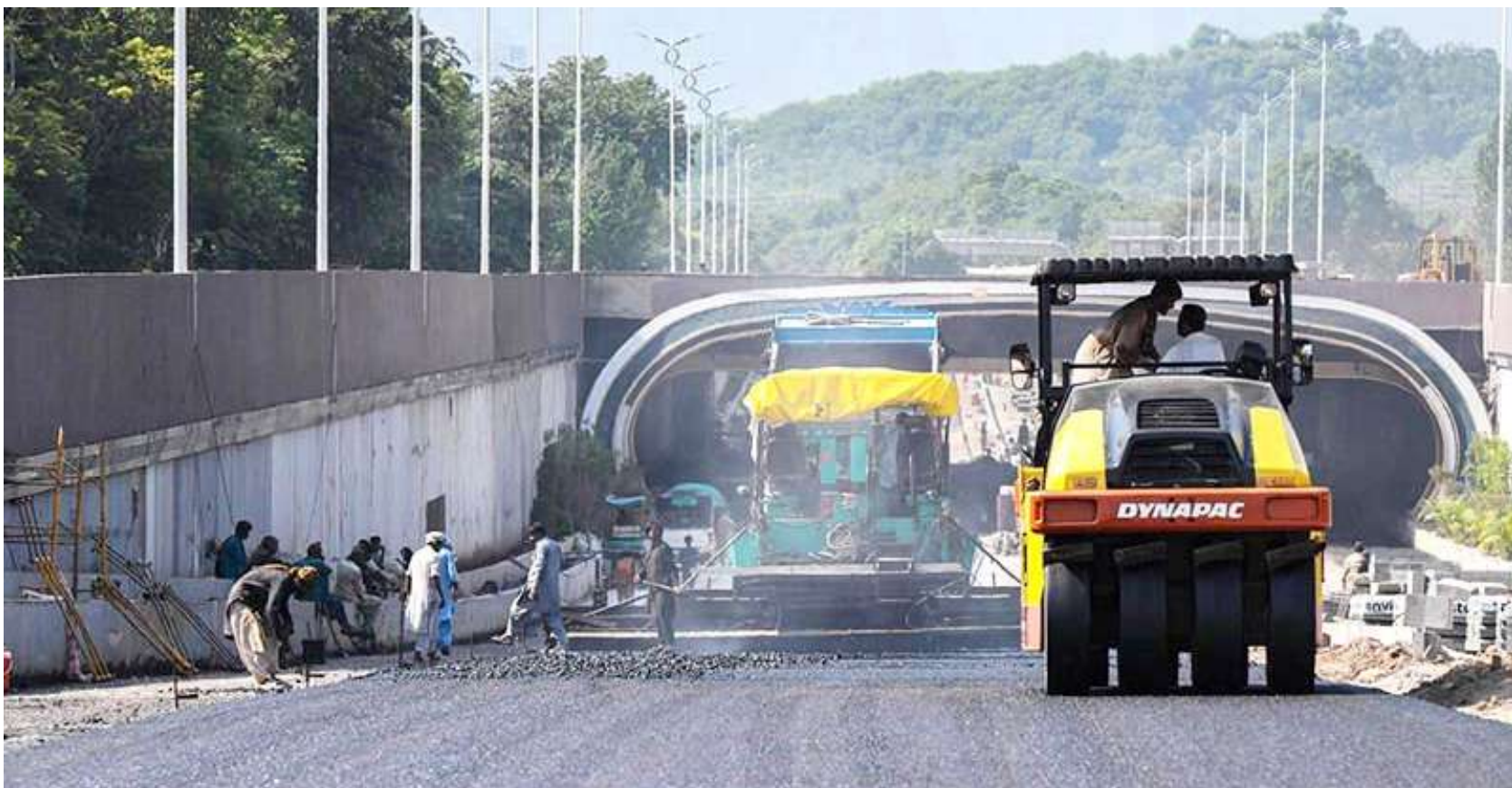
Heavy machinery and labourers work to complete the Park Road Underpass project, which is nearing completion.
