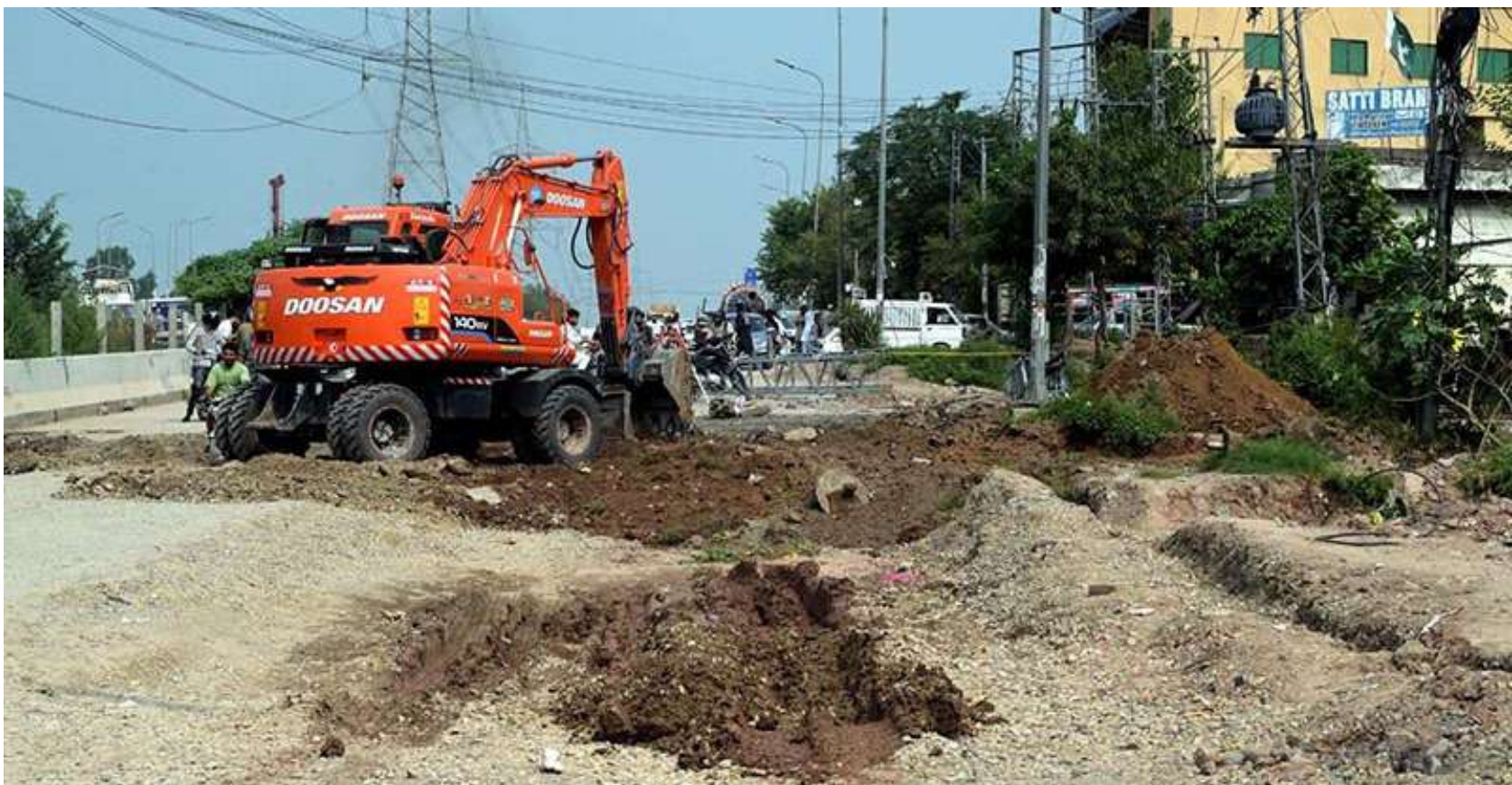
An excavator works on the construction of the service road extension along Expressway near Faizabad interchange.
