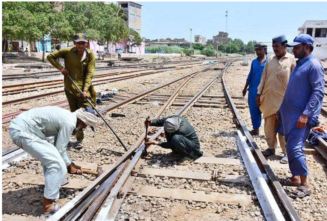
Railway workers are busy repairing railway tracks near Railway Station.
