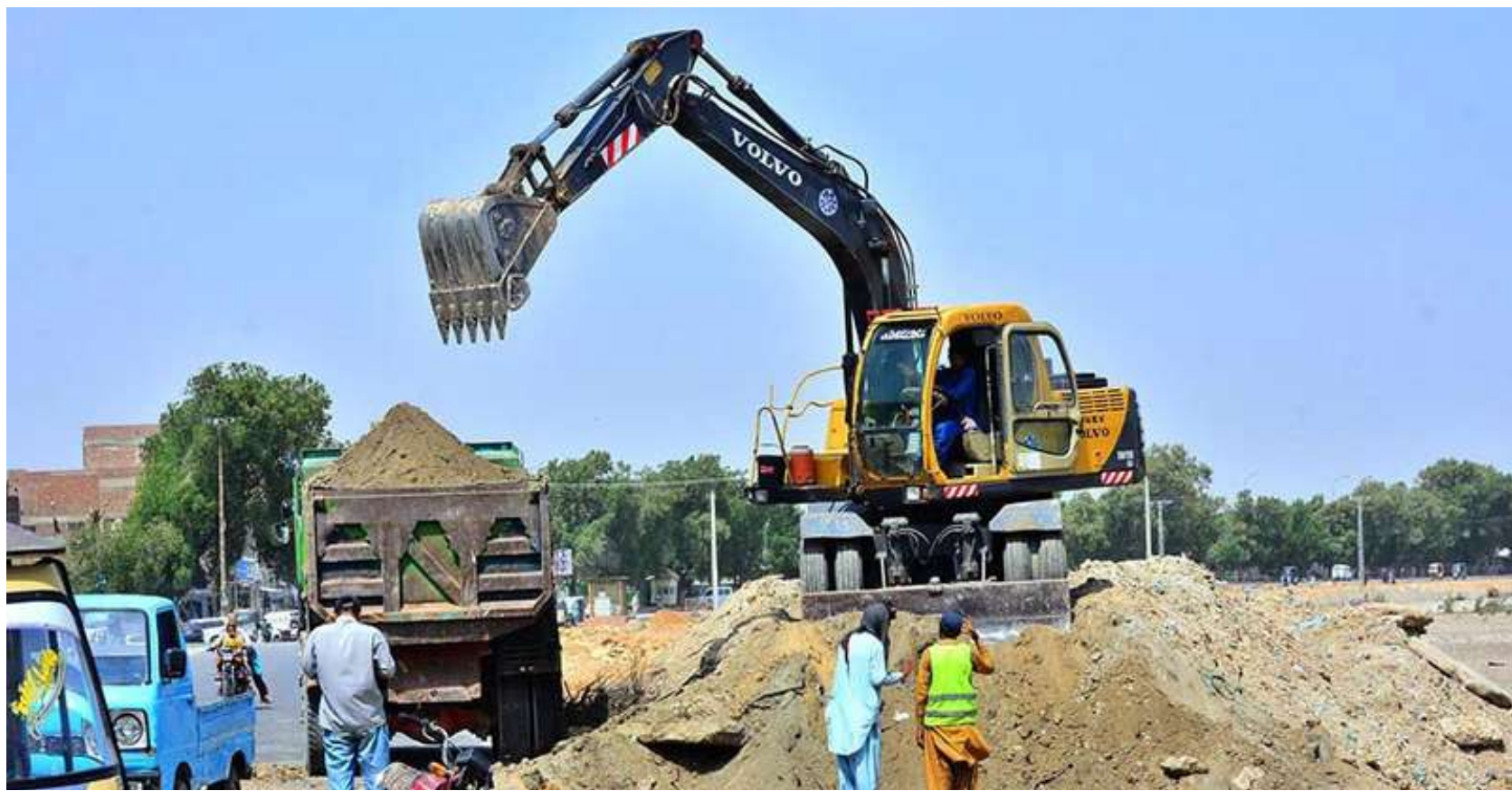
Labourers are busy construction work of new Wahduwah Road with heavy machine during development work in the city.
