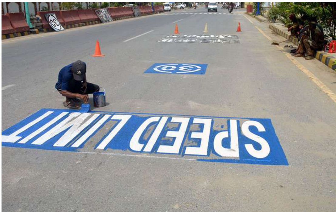
A worker paints road signs along Jail Road as part of routine maintenance work in the city
