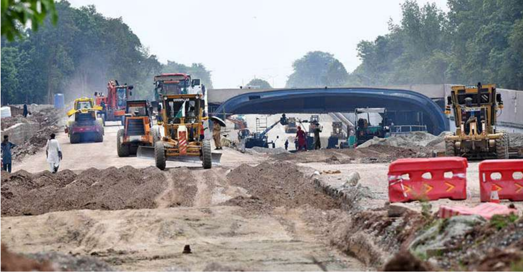
Heavy machinery is deployed at an underpass construction site along Park Road as development work progresses in the federal capital
